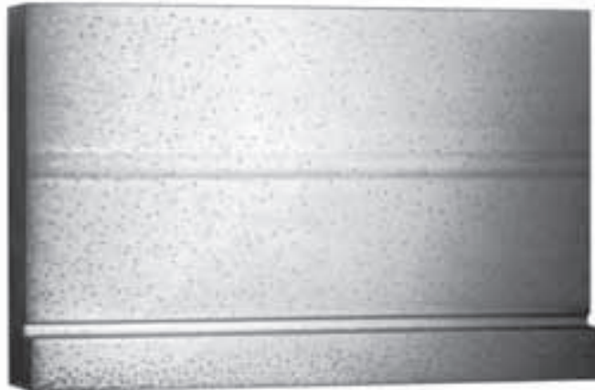
Typical appearance of corroded surfaces
